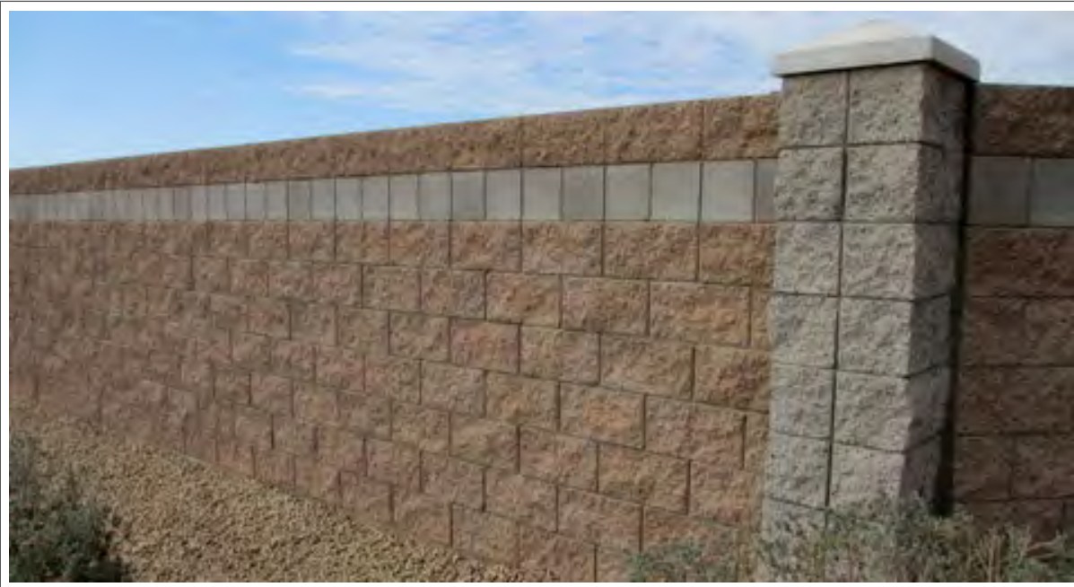
RESIDENTIAL BOUNDARY WALL
