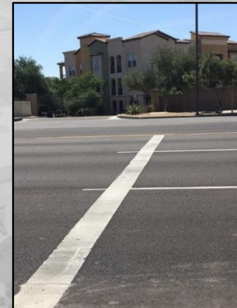
After Rehab Example (Reems Road)
