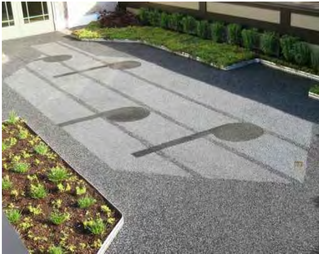
MUSICAL NOTES DECORATIVE PAVING 3 (SANDBLASTED INTO CONCRETE)
