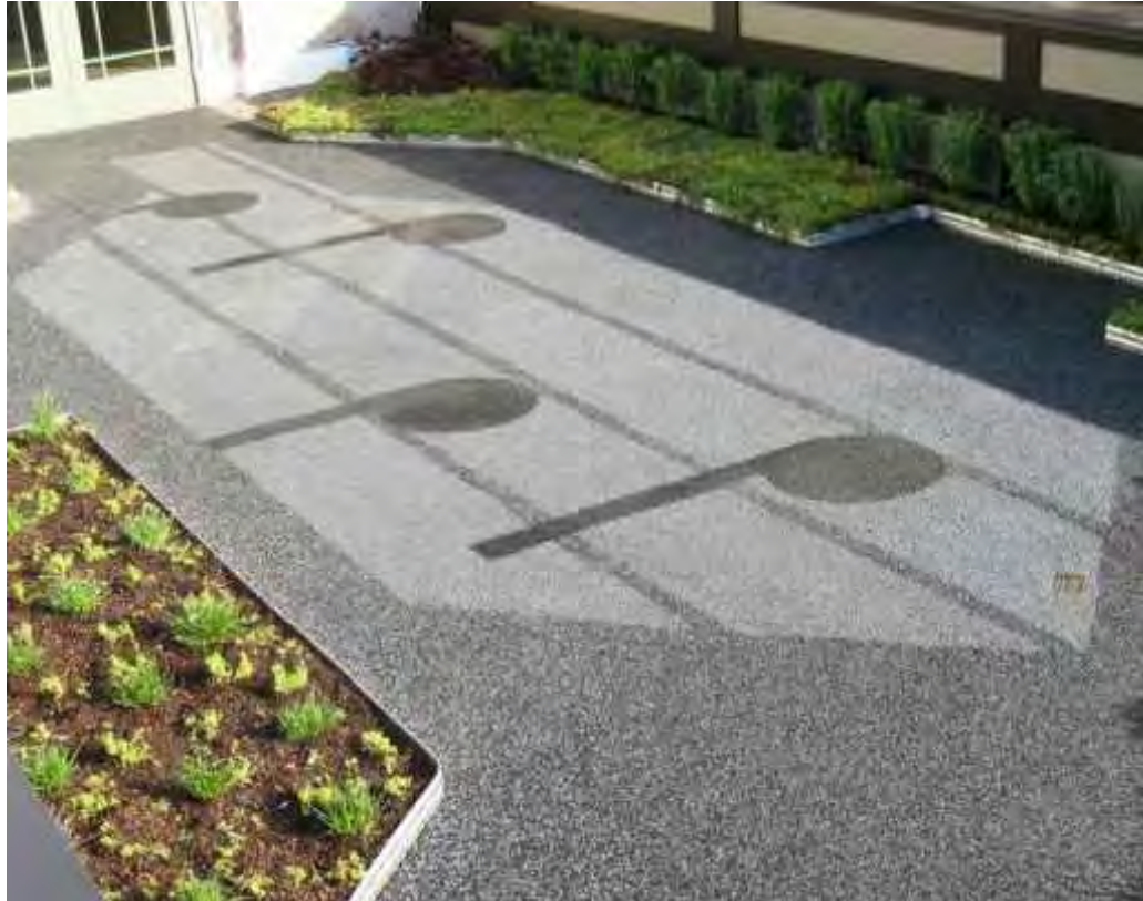
MUSICAL NOTES DECORATIVE PAVING 3 (SANDBLASTED INTO CONCRETE)
