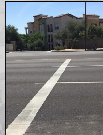
After Rehab Example (Reems Road)
