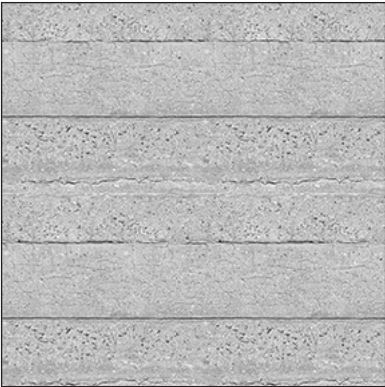
M-3 (Concrete) Board-Formed Cast In Place Raw Finish
