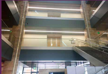
-2nd & 3rd Floor Walls
