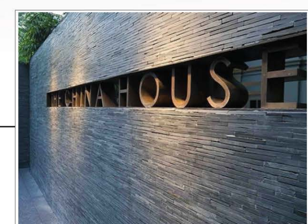
EXTRUDED STEEL SIGN BUILT INTO ENTRY MONUMENT WALL
