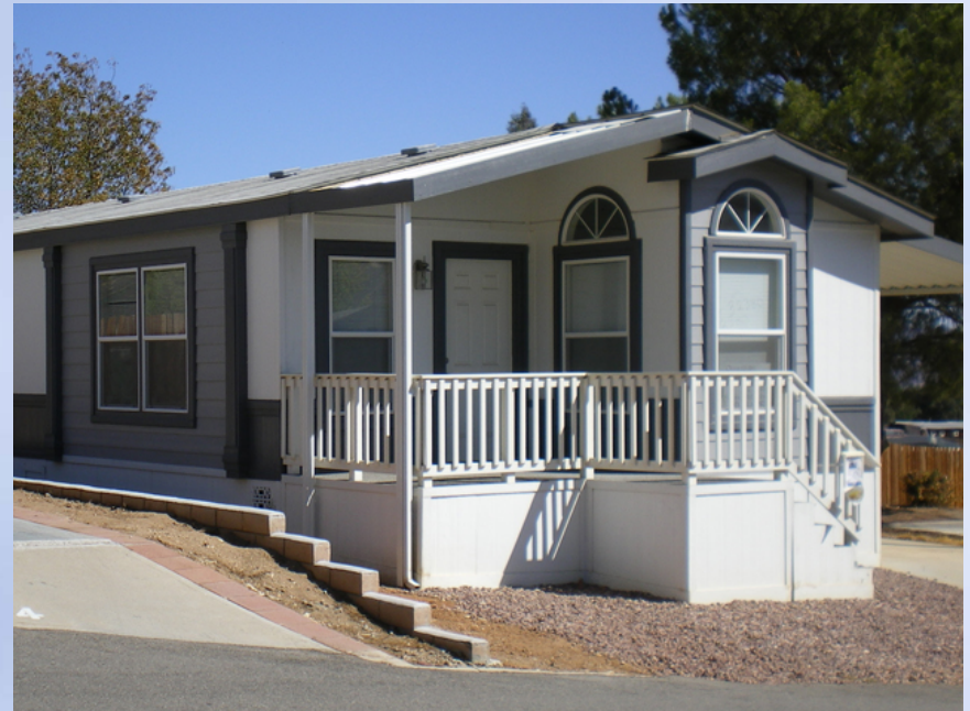
Even though it has steps, the architecture and the foundation do not resemble SHD built design requirements.
