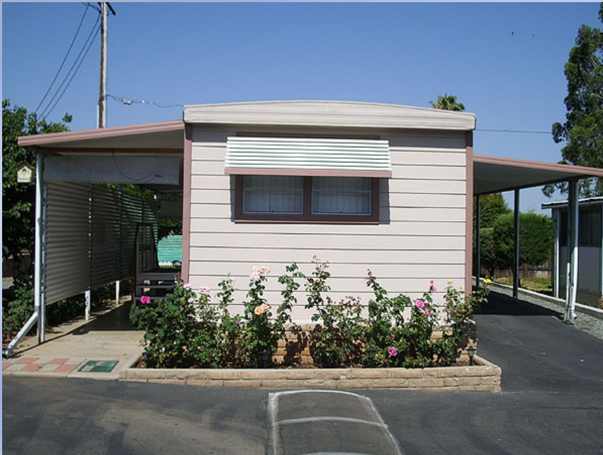
Even though it looks “newer”, the architecture and the design does not resemble SHD design requirements.
