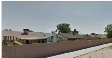
Example of unacceptable rear yard massing
