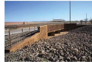
SIMULATED DESERT VARNISH & STANDARD FORMLINER ON VERTICAL CONCRETE
