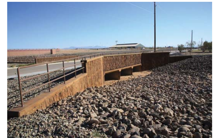
SIMULATED DESERT VARNISH & STANDARD FORMLINER ON VERTICAL CONCRETE
