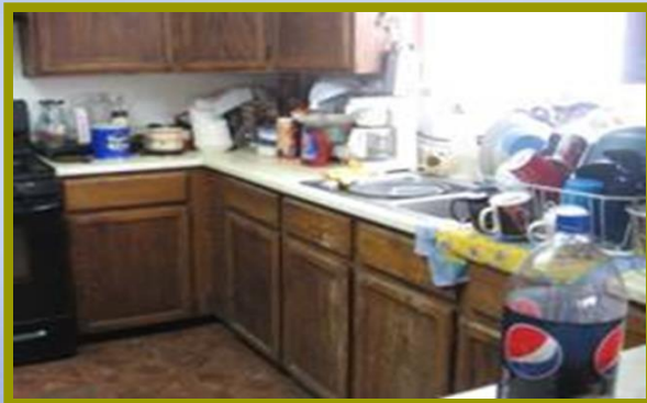
EMERGENCY REPAIR BEFORE
