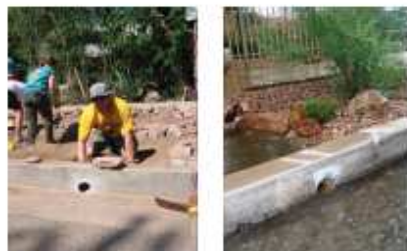
Curb Core Examples - 4" Diameter (Tucson Standard)
