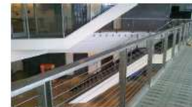
Double-plate post railing example
