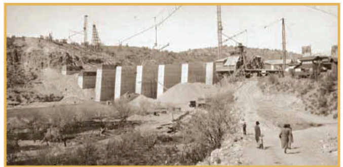
Frog Tanks Dam, now known as Waddell Dam, under construction in 1928. Courtesy of Maricopa Water District
