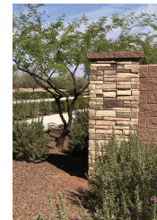
EXISTING WALL & COLUMN
