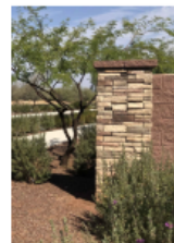
EXISTING WALL & COLUMN
