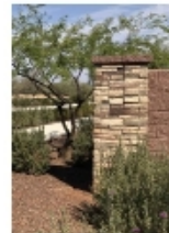
EXISTING WALL & COLUMN
