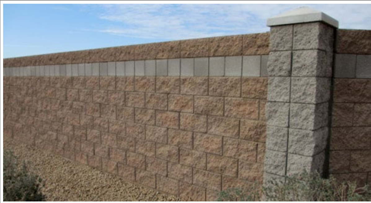
RESIDENTIAL BOUNDARY WALL
