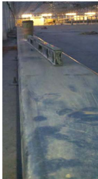
Completed rail system
