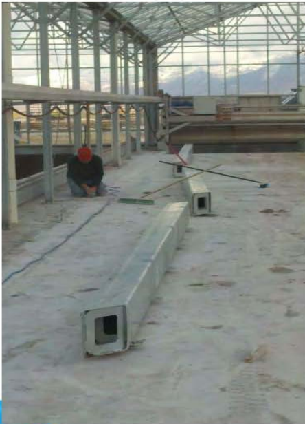
Galvanized Steel Rails - ~20ft segments
