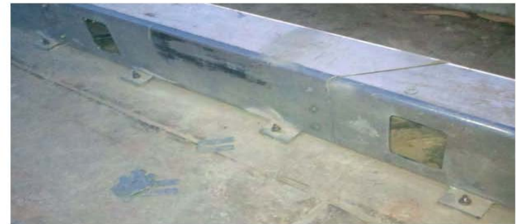
Steel Rail Connection point -anchored to concrete floor, leveled with shims,
