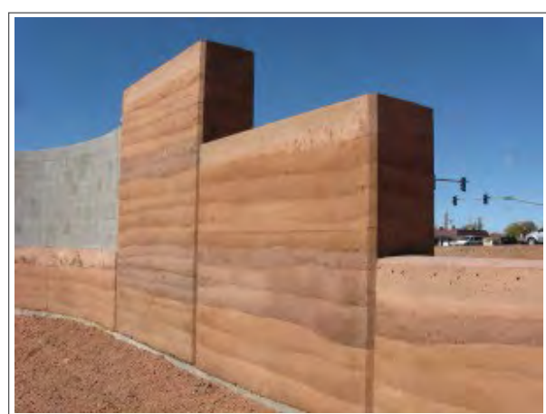
RAMMED EARTH WALLS
