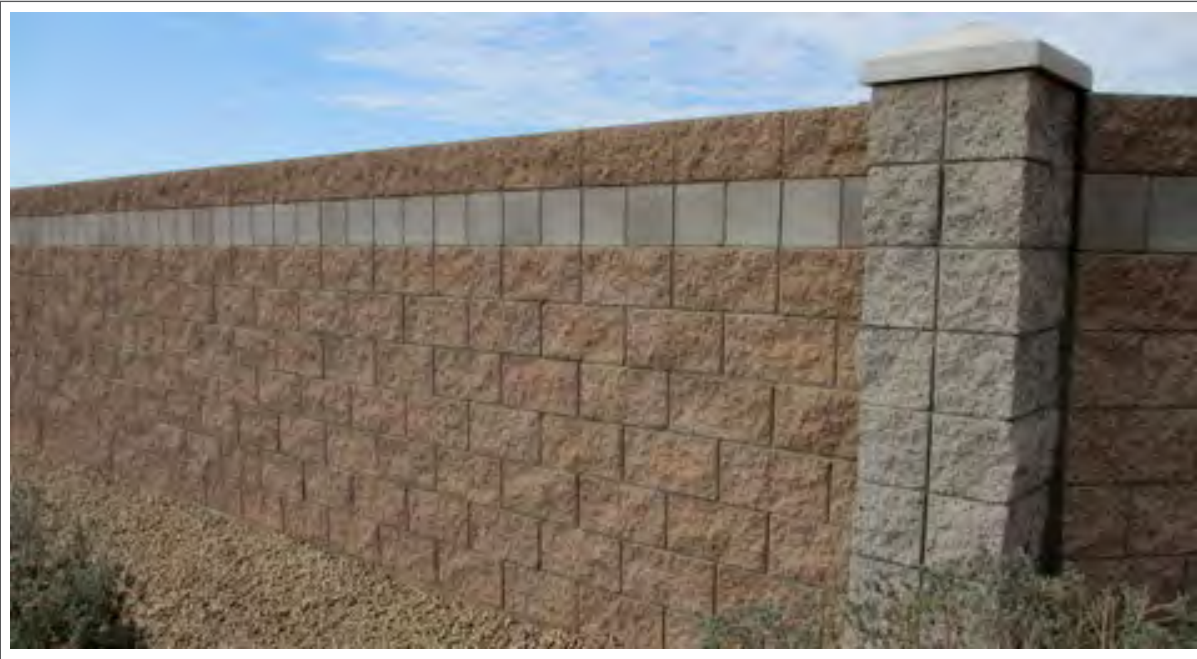
RESIDENTIAL BOUNDARY WALL
